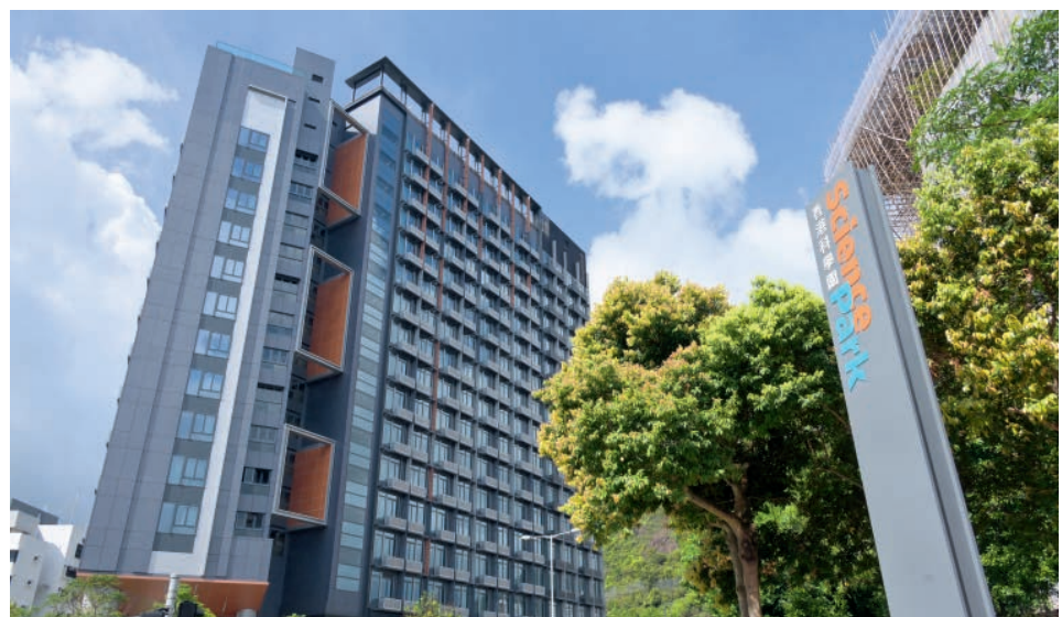
The InnoCell at the Hong Kong Science Park provides around 500 residential units to its R&D personnel as a living and co-creation space.
